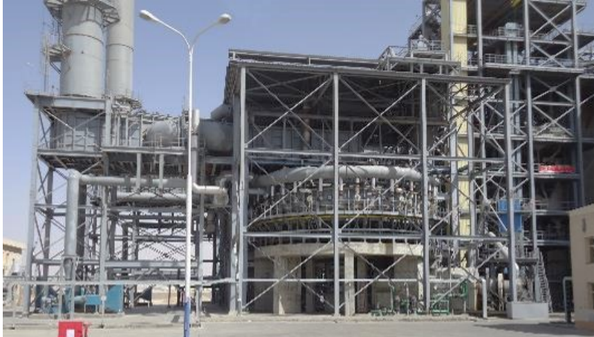
Figure 1. Rotary hearth furnace calciner, ©TenoVA.
